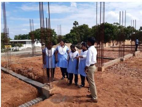
II year Civil Engineering students observing the design of building structure during industrial visit
