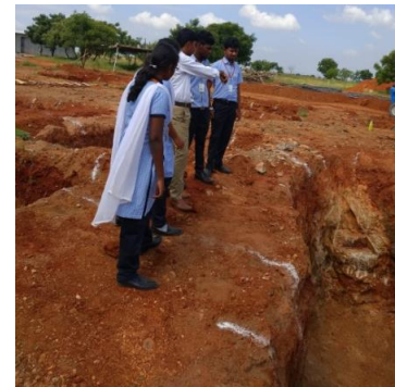
Civil Engineering students exploring on earth excavation techniques during industrial visit
