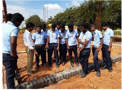
II year Civil Engineering students observing the safety points in construction during industrial visit
